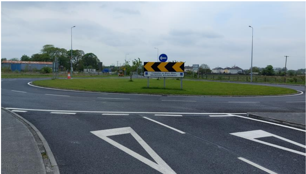
FIG.2 – BAUNMORE ROUNDABOUT RE-SURFACING
